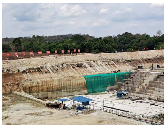
Kidunda dam (Tanzania) under construction
