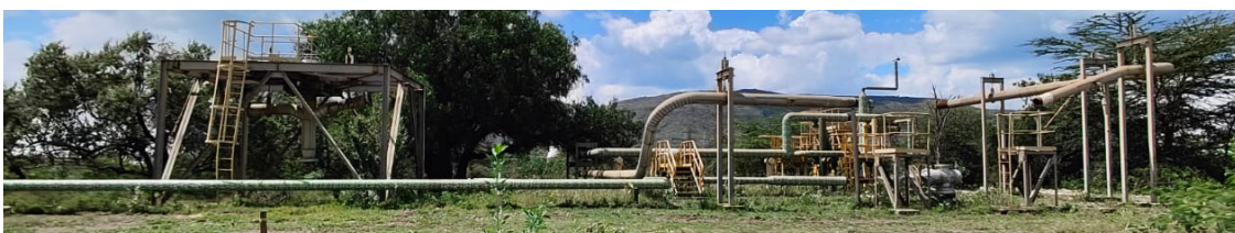
Geothermal Infrastructure in Hells Gate National Park, Kenya
